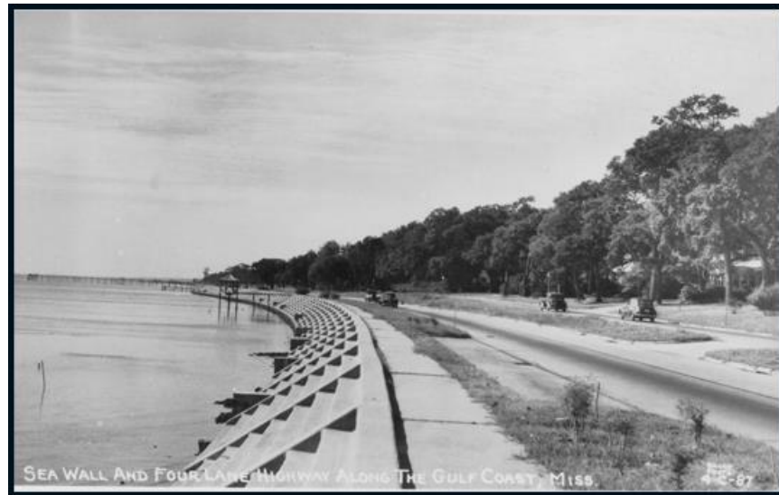
Figure 1.4 Harrison County Seawall circa 1942
